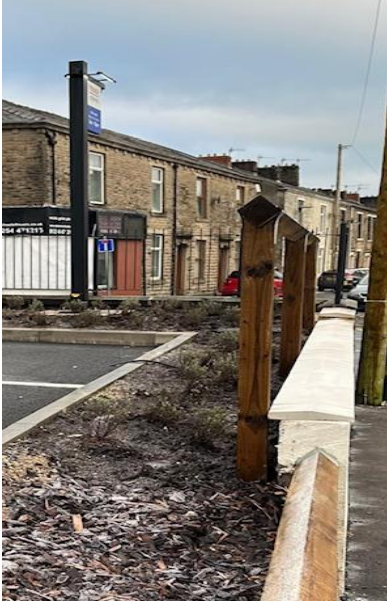
Knee high fence running into rendered wall not level
