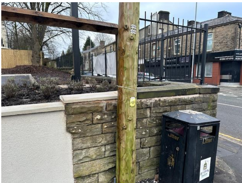
Knee high fence running into rendered wall not level
